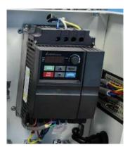
**Delta VFD**. The VFD-EL series is multiple function new generation micro type AC drive. It has built in EMI filter, RFI switch, easy DC bus sharing for side-by-side installation, high precision current detection, overload protection, and a built In keypad
